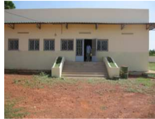
Newly built IER biotechnology building in Sotuba, Mali
